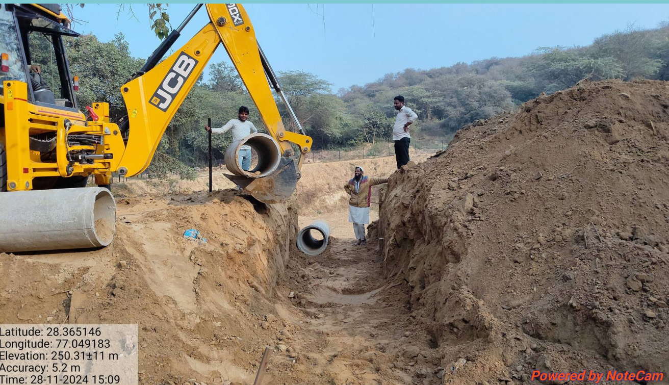
SURVEYING THE SLOPE
