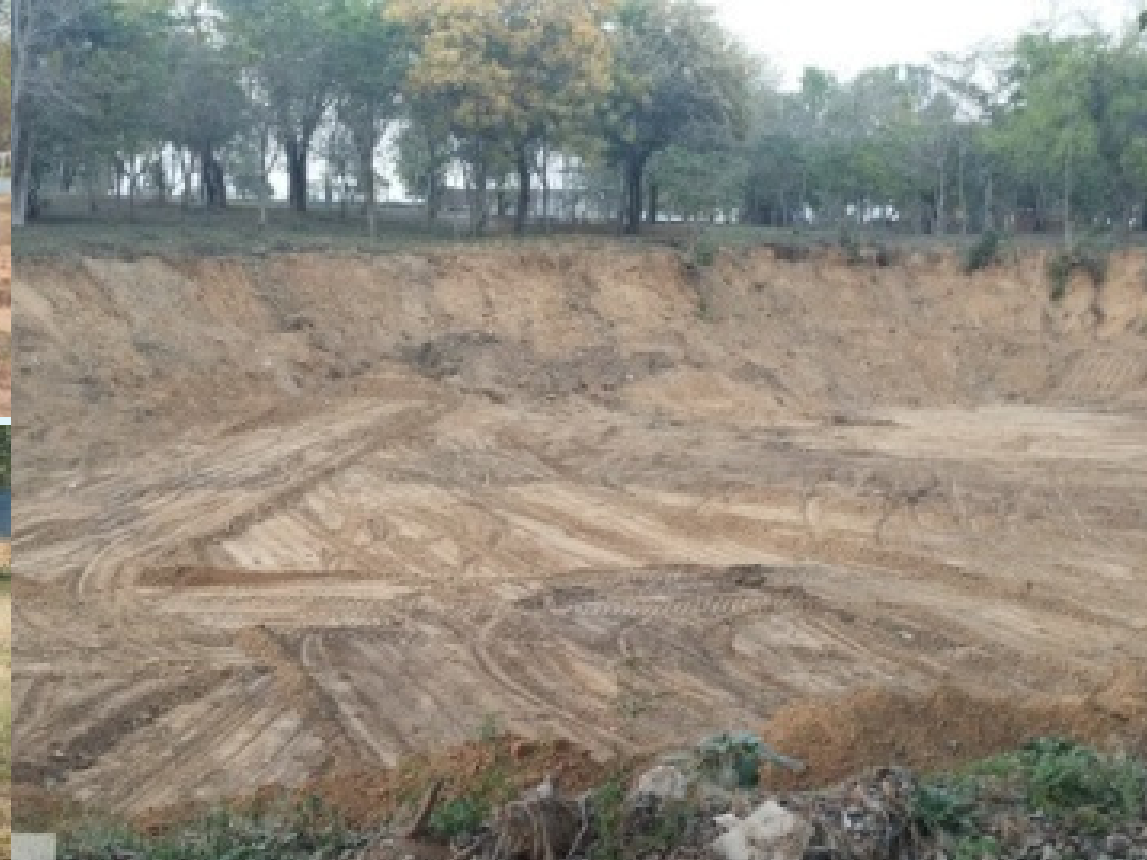
POND DREDGING + PROFILING
