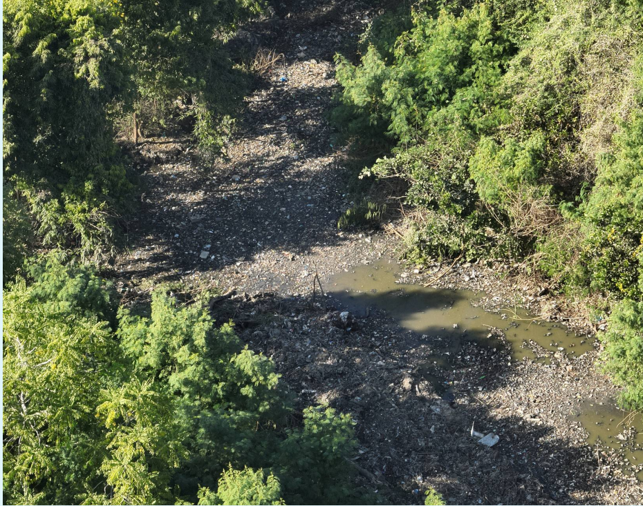
Clogged channel Uncontrolled polluted runoff Damaged drain walls
