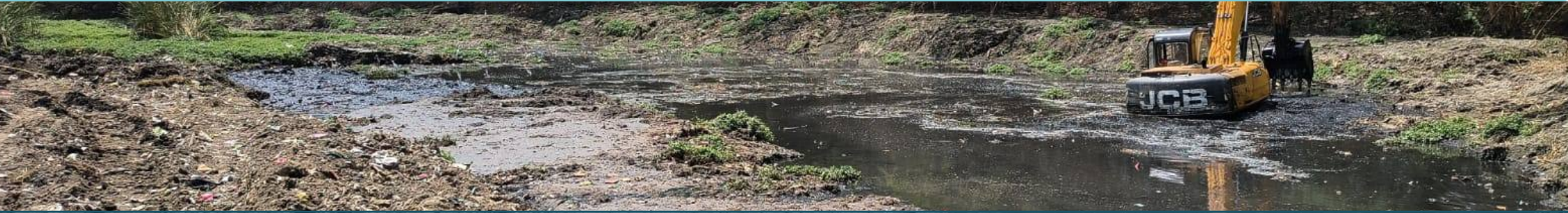
Desilting of pond
