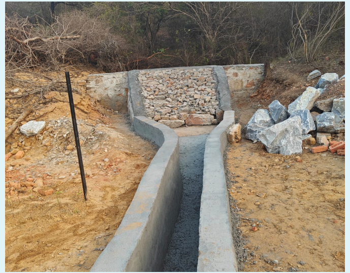
Figure: Gully Plug for Soil & Water Conservation
