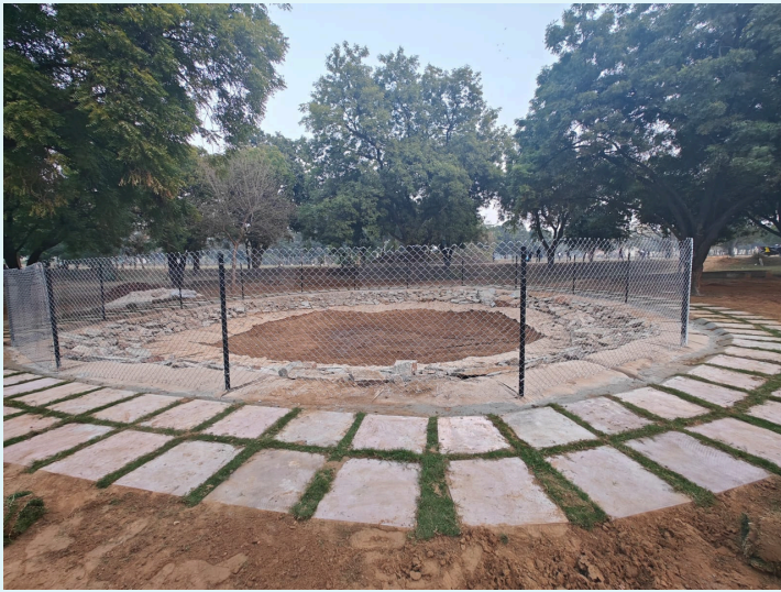
Figure: Detention Pond
