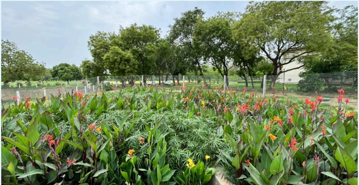
Figure: Anaerobic Baffled Reactor with vegetated gravel wetlands
