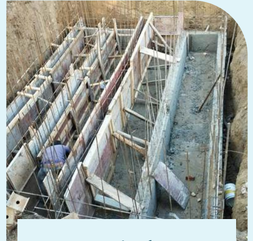
RCC Work of WWTP
