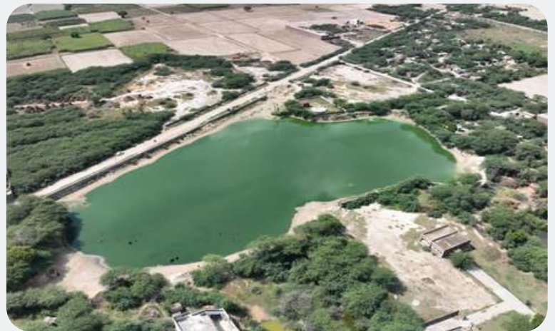
Drone image of Pond before Intervention
