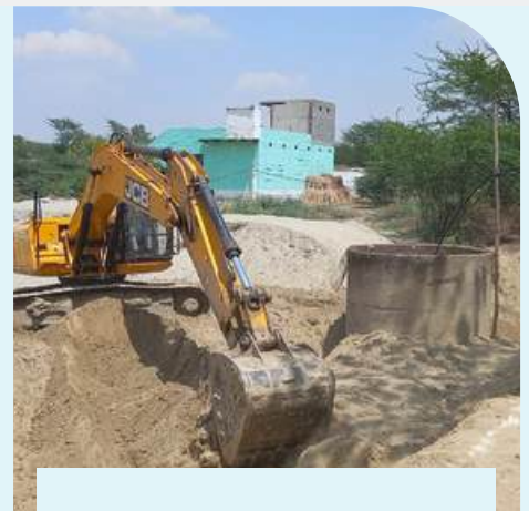
Leveling of the site
