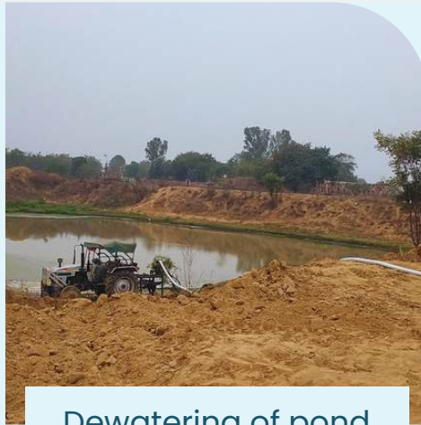
Dewatering of pond
