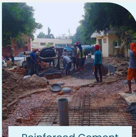
Reinforced Cement Concrete Casting Work
