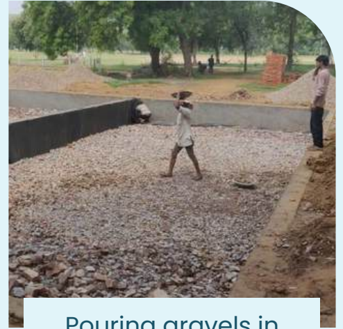
Pouring gravels in wetland
