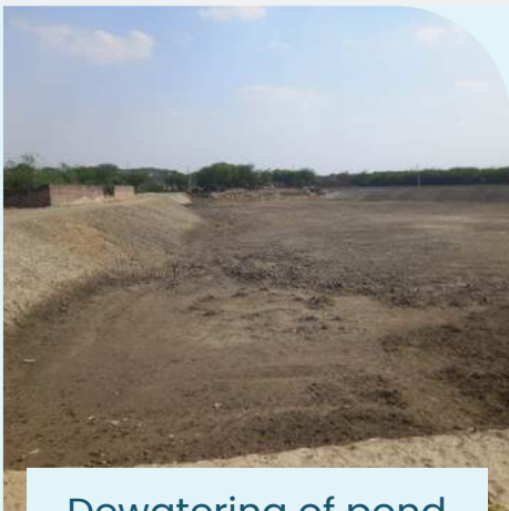
Dewatering of pond
