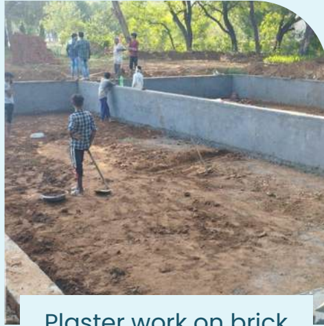
Plaster work on brick walls of constructed wetland
