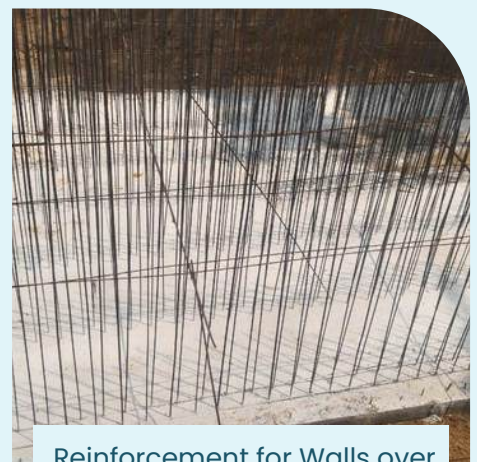
Reinforcement for Walls over the Raft Foundation of WWTP
