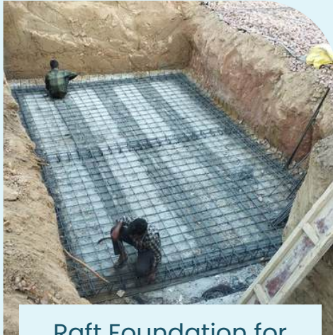
Raft Foundation for WWTP
