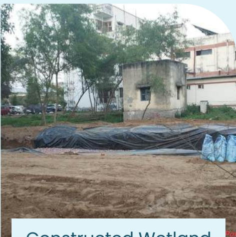
Constructed Wetland Development
