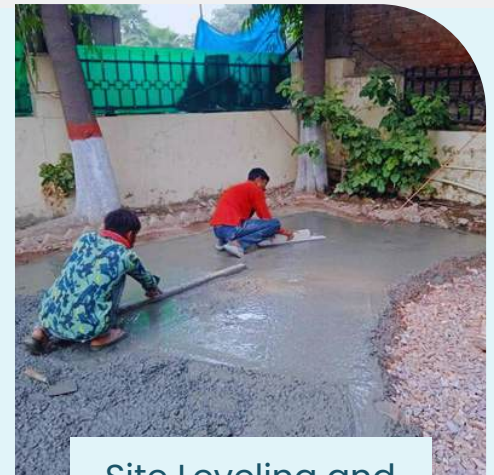
Site Leveling and Surface Finishing
